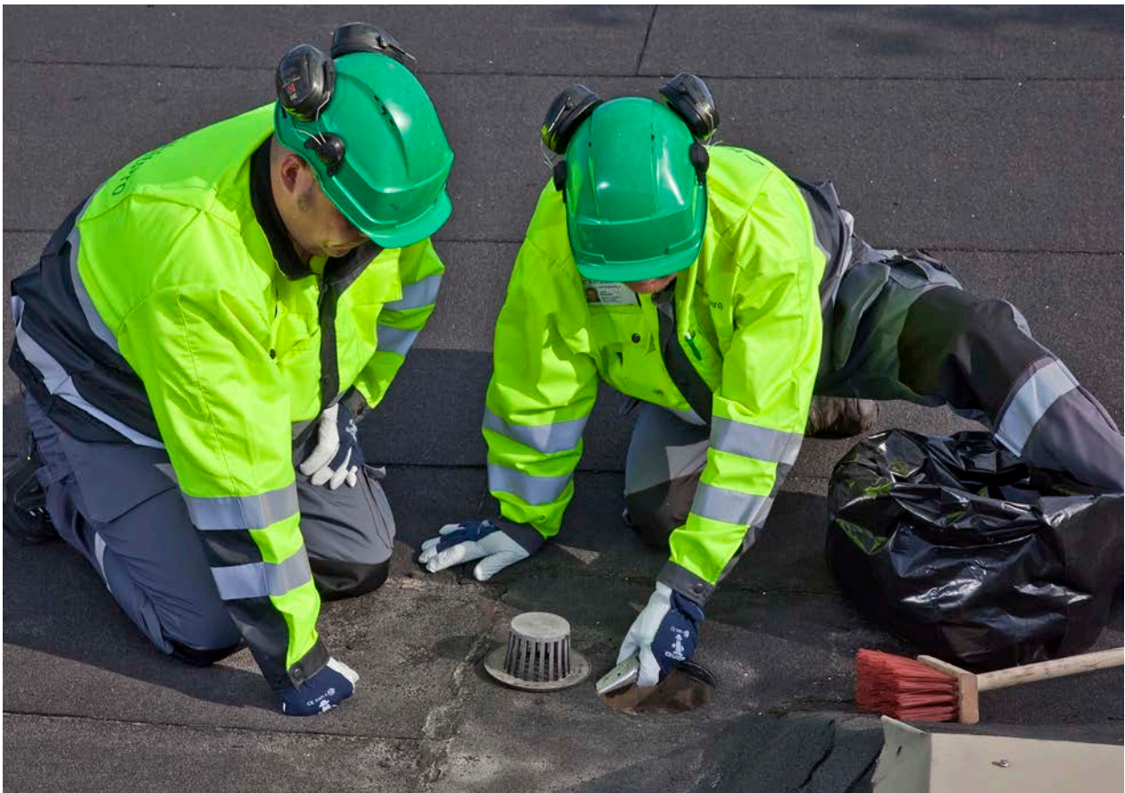
When waterproofing with bitumen, all the details on a roof may be made waterproof in a simple way.
