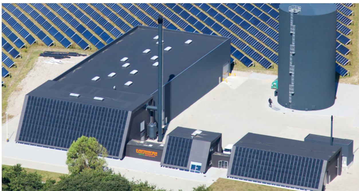
Gråsten solar plant in Denmark.
