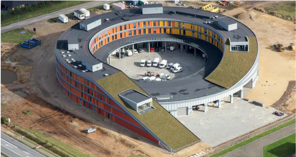
Innovest in Skjern is a building that includes activities with focus on education, business and innovation. On 1,000 square meters of the roof there is a customised version of green roof, Nature Impact Roof.
