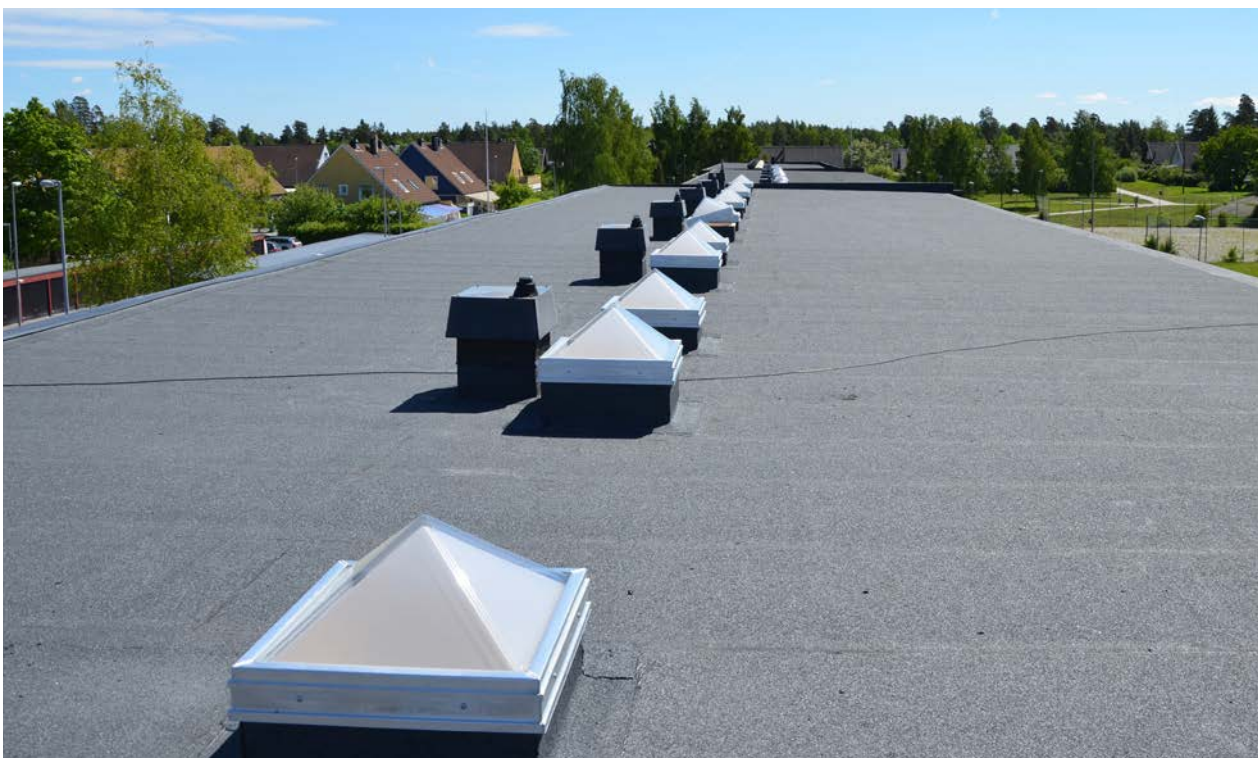
Domes or roof lanterns are the best solution for letting in light in the middle of buildings with flat roofing.
