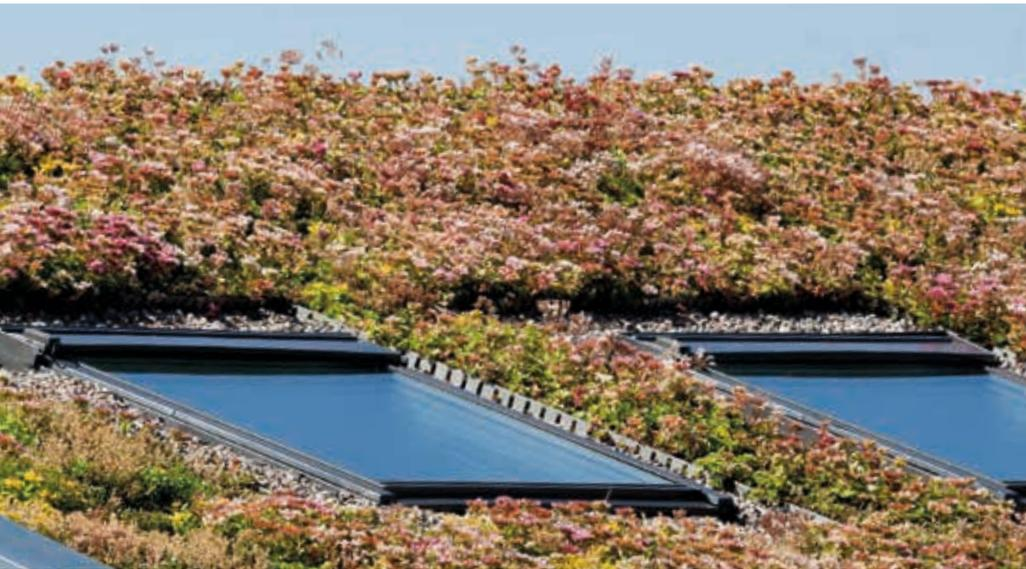
Sedum is a durable plant blend for low-incline roofs and is decorative while offering a number of environmental benefits. At the same time, good preparation with a high-quality sealing membrane is required to guarantee the roof's protective function. Nordic Waterproofing offers a range of products for green roofs.
