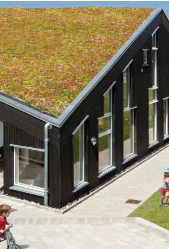
The "Solhuset" kindergarten in Hørsholm, Denmark has an area of 1,300 m<sup>2</sup> and was constructed based on an "Overactive House" concept. Several different construction companies worked together to develop a building that meets all of the requirements that can be imposed on a positive environment for children, at the same time as the building produces a surplus of energy. Taasinge Elementer has supplied different solutions for roof and wall components for Solhuset.
